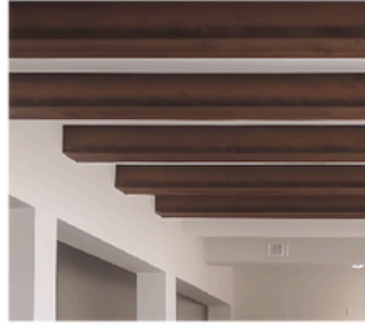
Ceilings White flat Drywall with wooden beams
